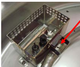
Pilot Window lined up with burner hole.
